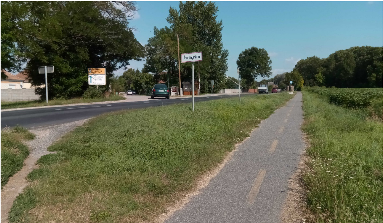
High-quality cycle path, but the maintenance could be improved to prevent the edges from being overgrown.
