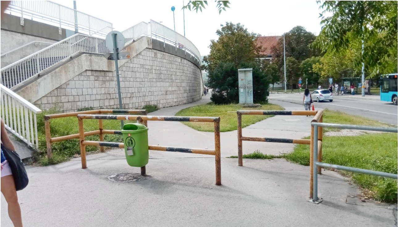
Example of a chicane that is difficult to pass with a tandem or trailer.
