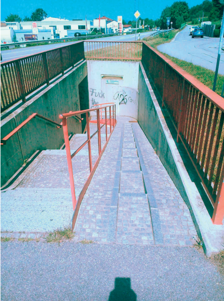
Stairs with ramp but barely visible sign close to Passau (section 12). Dark underground passage could also be a social safety challenge.
