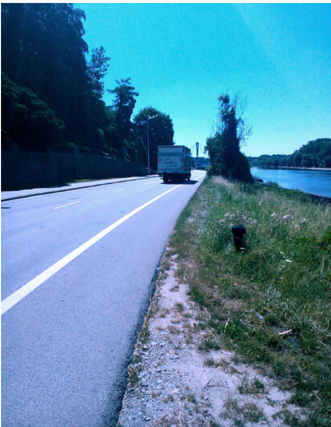
Very high traffic on public road close to Deggenu (section 11). Painted cycle lane/paved shoulder with width of less than 1.5 m.
