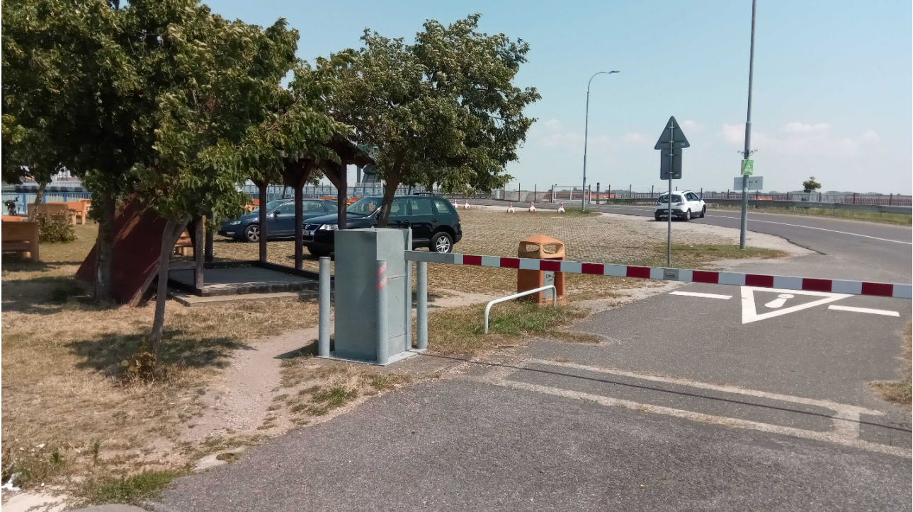
One of the barriers that need to be adapted to meet the Additional European Certification Standard criteria.
