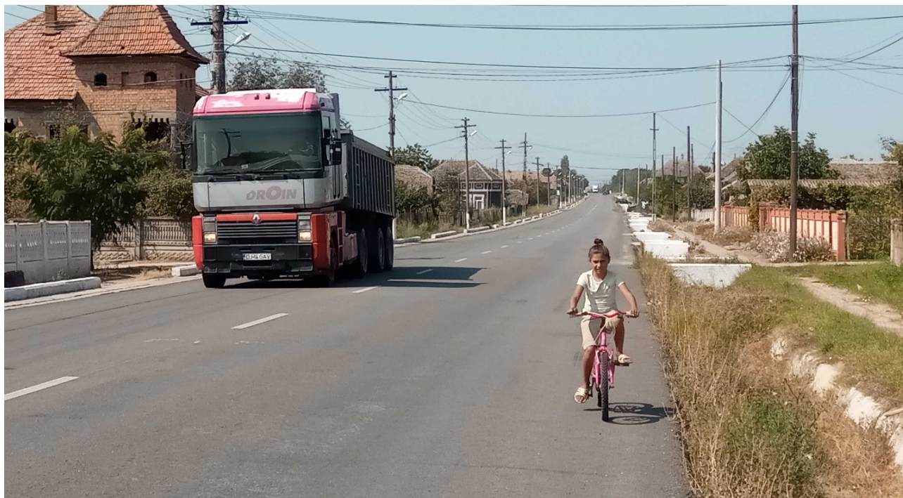
In many locations, the construction of a cycle path would improve also safety of local inhabitants. Basarabi near Calafat, daily section 69.
