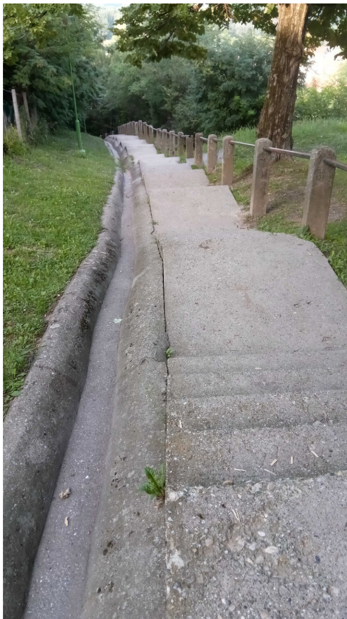
Stairs in Ilok. To consider whether they should be a part of the EuroVelo route.
