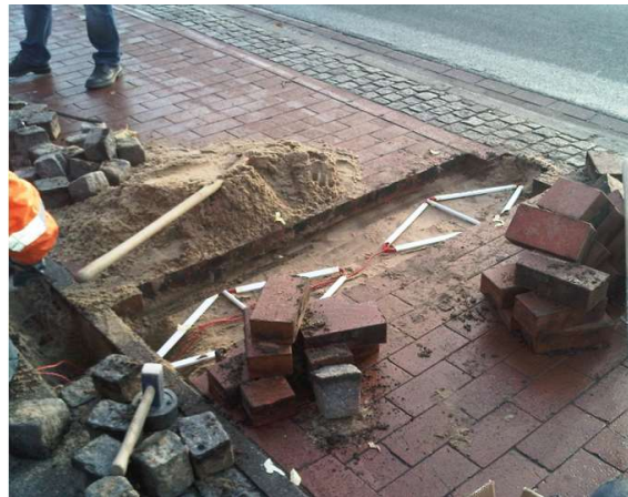
Figure 3 Inductive loops under paving, source: Eco-Counter
