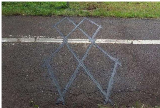
Figure 1 Inductive loops on asphalt, source: Eco-Counter
