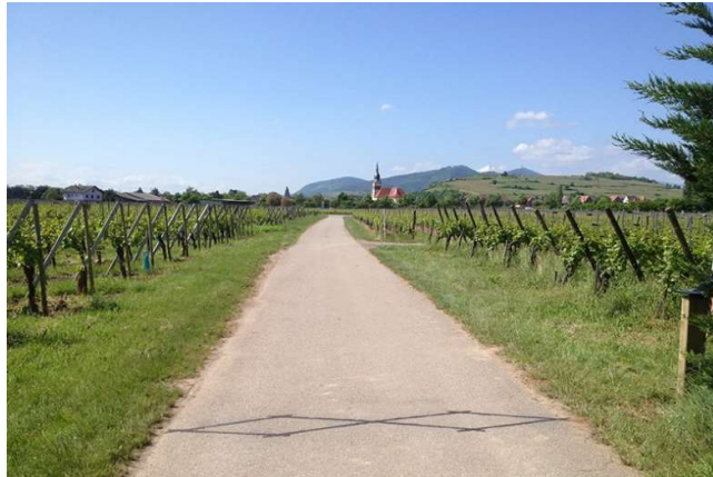
Figure 7 Inductive loops on greenways (pedestrians, bicycles), source: Eco-Counter
