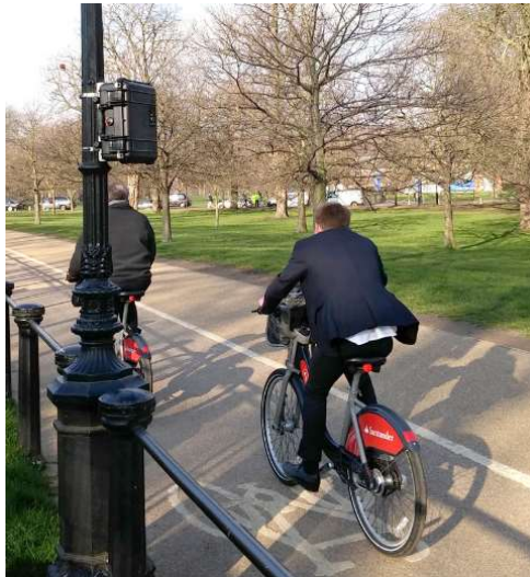
Figure 7 Radar installed at the pole, source: CA Traffic
